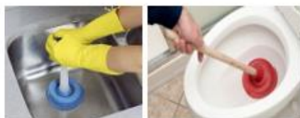
Unblocking a basin, sink & toilet
