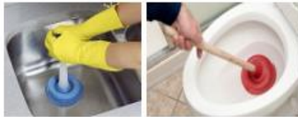
Unblocking a basin, sink & toilet
